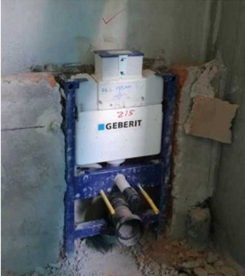
Pre-wall installation with drywall construction and solid rear wall connection
